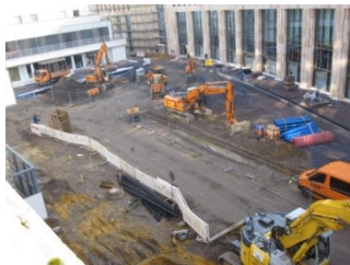
A grandstand view over the building site from our balcony ...
