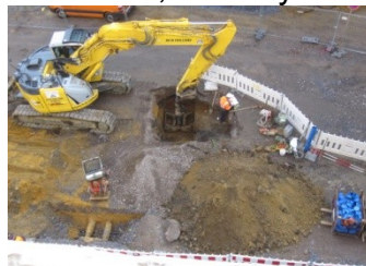
Excavating a manhole position with a grab ...
